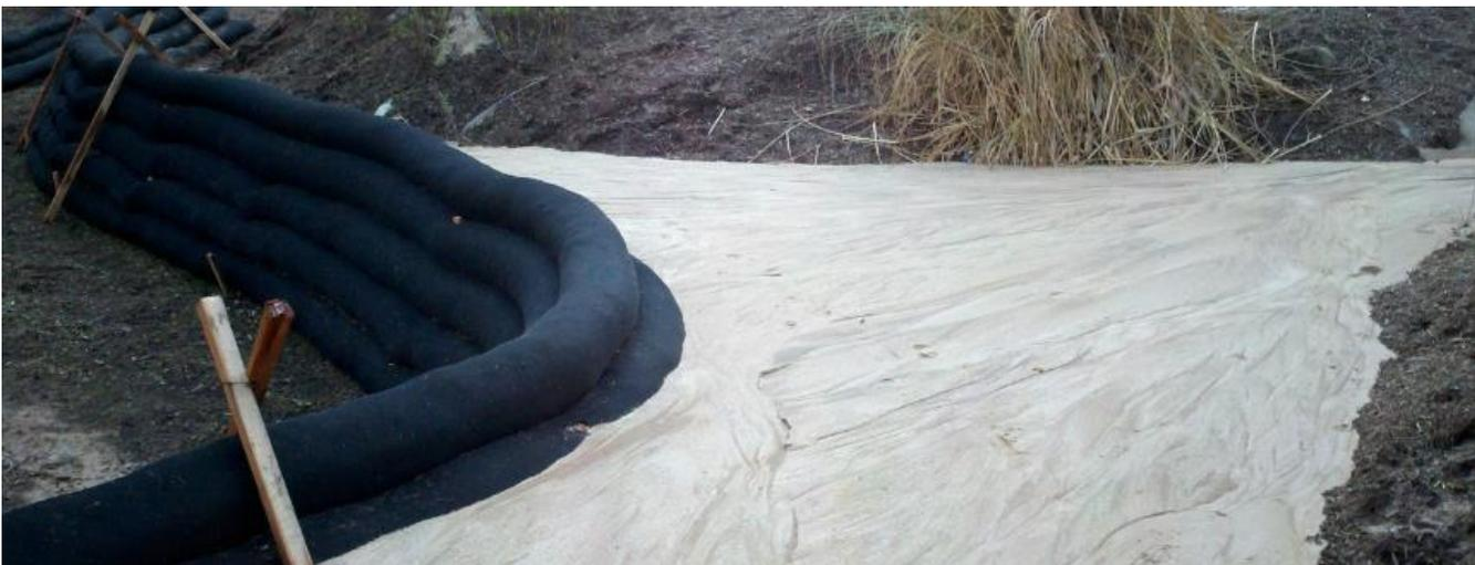
Sediment trap, 12-inch diameter filter socks in pyramid stack, photo courtesy of Filtrex
