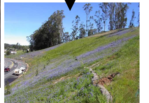
Picture: Erosion control measures
